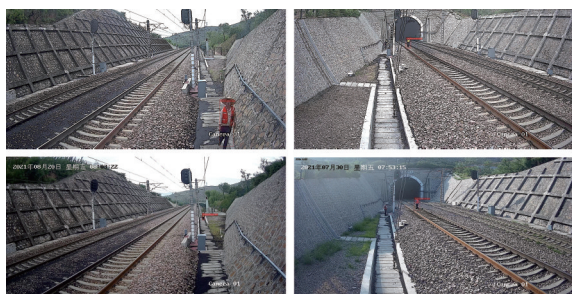
Fig.11 Several alarm images
