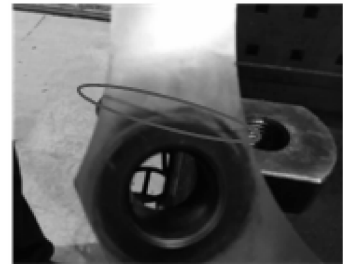
(a) Membrane fatigue crack
