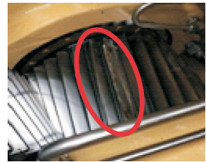
Fig. 12 Wear on gear system [31]
